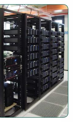
The dedicated cluster room has 1400 sq. ft. of usable floor space and is cooled by four 26-ton air conditioning units. Heat is transferred to a water/glycol mixture which is circulated to dry the rooftop coolers.
